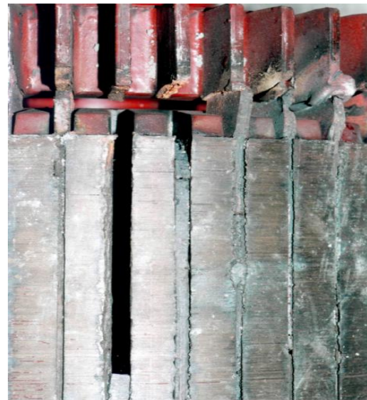
Fig. 1. The faulty cage with several cracked and broken rotor bars
